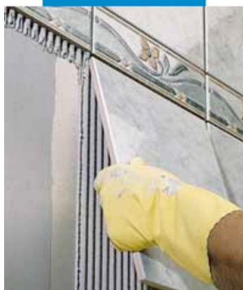
Installation of single-fired tile on wall render
