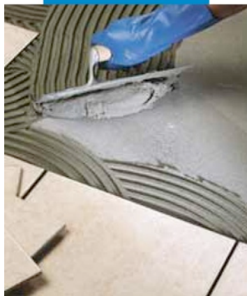
Installation of single-fired tile on floor
